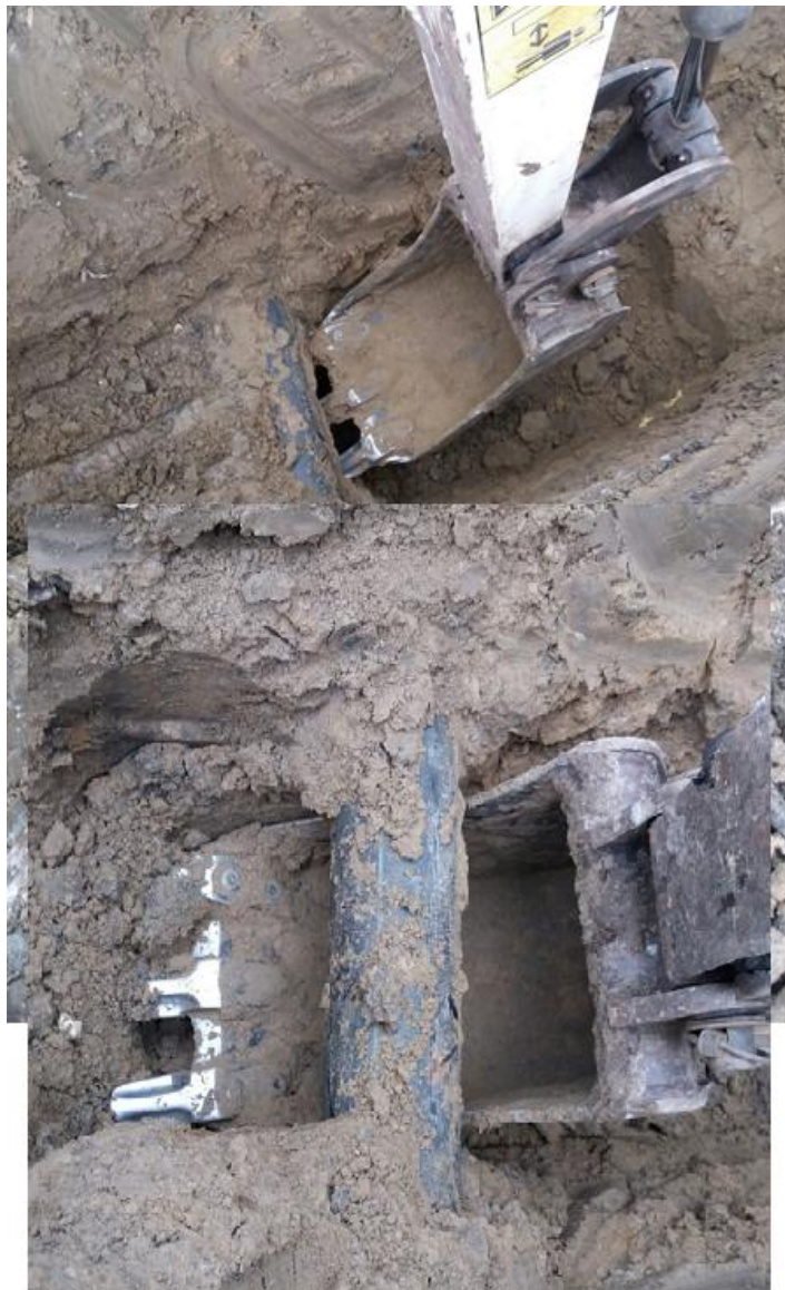
Fig.1. Actual situation of accidentally applying stress on the PE 100 polyethylene pipe by the excavator bucket
